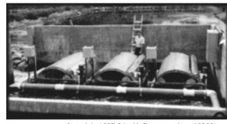
3 models 1607-24 with flow capacity = 16000 gpm
